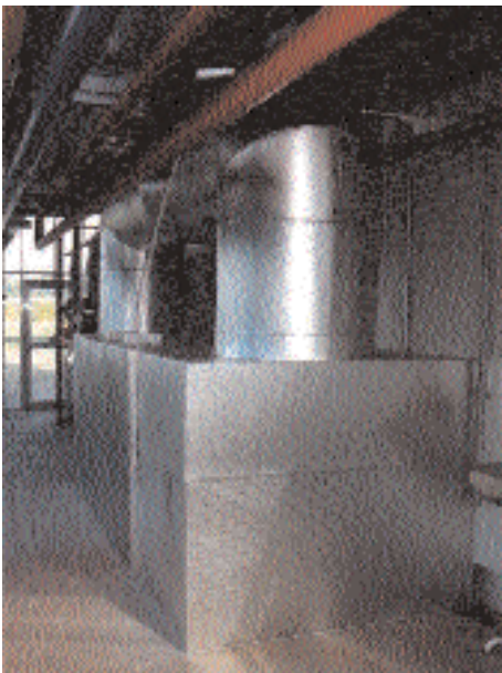
Fully Insulated ECO 2 PRO Reactor Housing (1 MW Unit) horizontal arrangement
