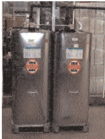
Modular Urea Storage Battery Tank 2 x 1 m 3 Capacity, Double Wall Design
